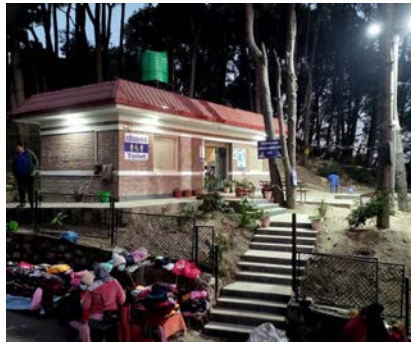
Public sanitation facilities. An Aerosan toilet center in Kathmandu, Nepal serves nearby market customers and is clean and well lit (photo by AeroSan).
