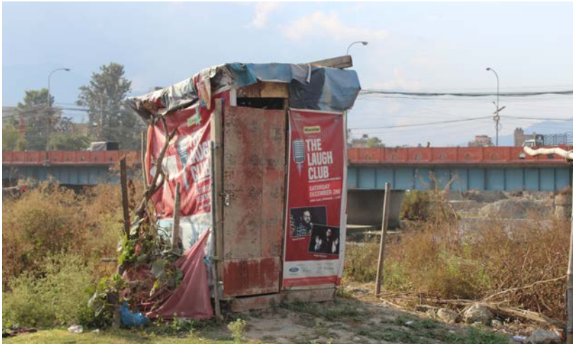
Lack of access to sanitation. Residents of Thapathali informal settlement in Kathmandu use a makeshift toilet (photo by Lakpa Sherpa).
