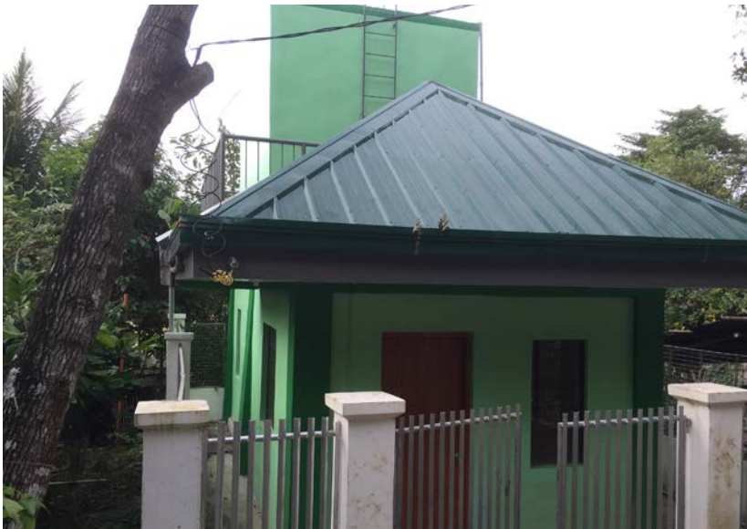
Community-led project in Janiuay. A rainwater harvesting and storage tank, and cooperative office, constructed in 2021 complement the community-managed water supply system in the village of San Julian (photo by Philippine Rural Reconstruction Movement).
