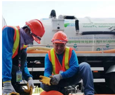
Sanitation services. Laguna Water Staff emptying a septic tank in Laguna, Philippines (photo by Laguna Water).
