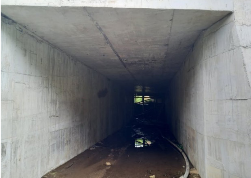
Community-led project in La Trinidad. Climate-resilient concrete box culverts for flood risk reduction were constructed in three key sites in the village of Betag in 2021 (photo by Philippine Rural Reconstruction Movement).
